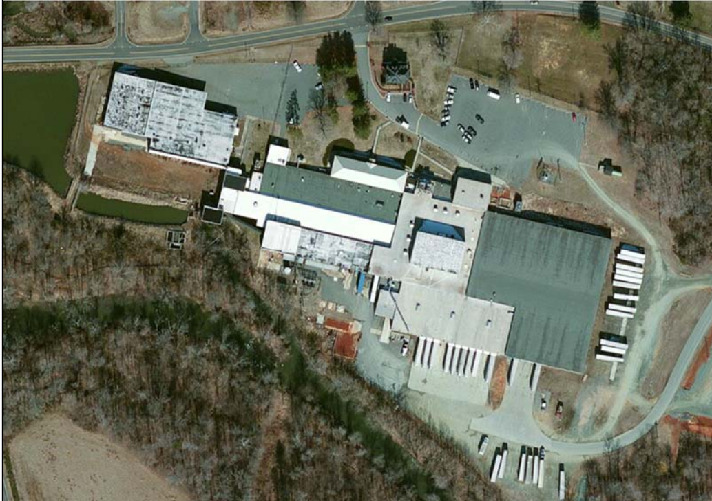
Figure 14: Altamahaw Cotton Mill, aerial view from 2010 with north half of west section standing
