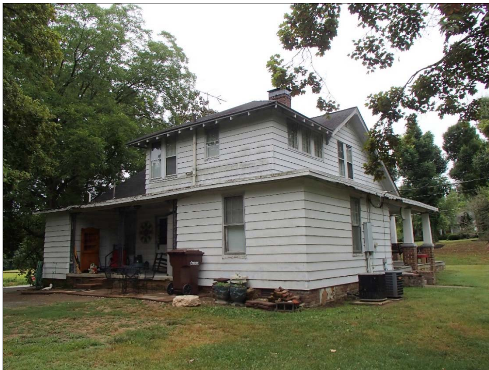
Figure 37: Simpson House, southwest corner
