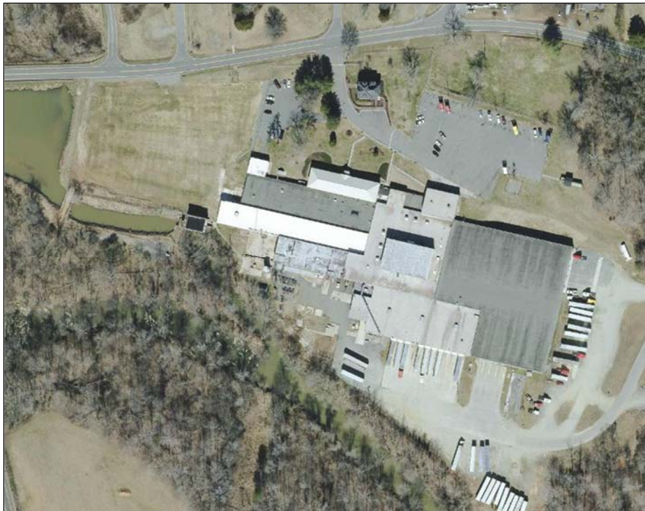
Figure 15: Altamahaw Cotton Mill, aerial view from 2014 after demolition of western section
