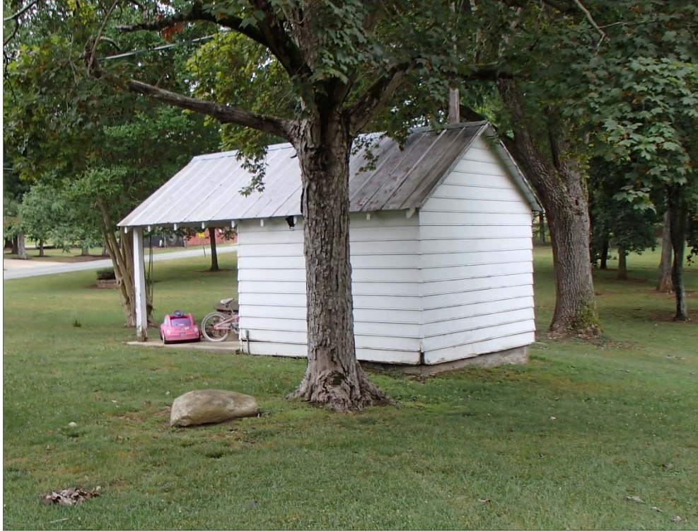
Figure 44: Simpson House, well house, northeast corner
