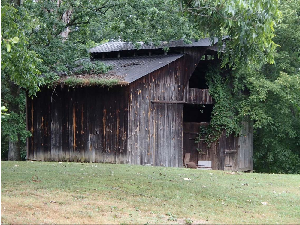
Figure 40: Simpson House, barn, south corner
