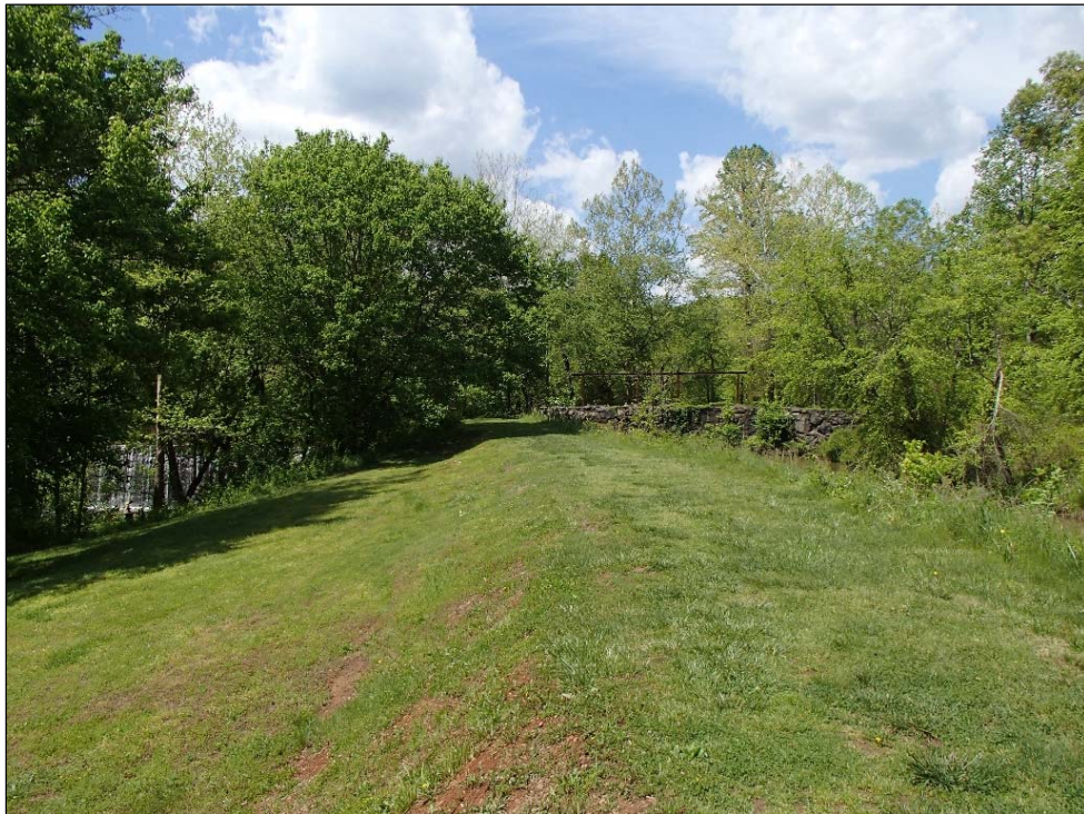
Figure 19: Altamahaw Cotton Mill, berm between Haw River dam (left) and sluice gate dam (right)
