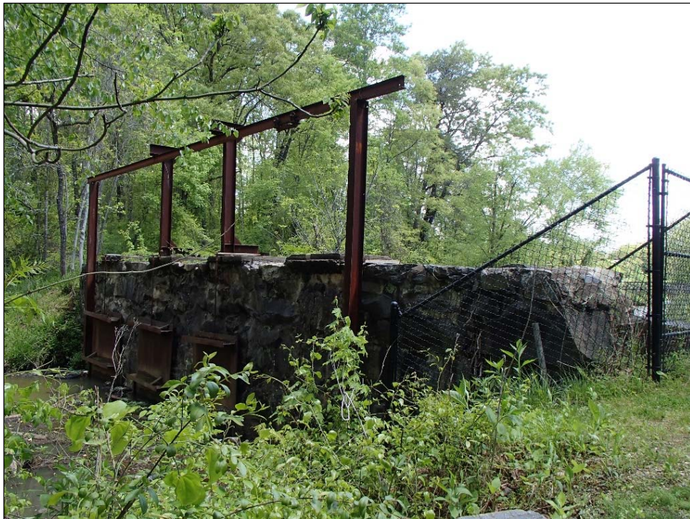
Figure 23: Altamahaw Cotton Mill, sluice gate, west elevation
