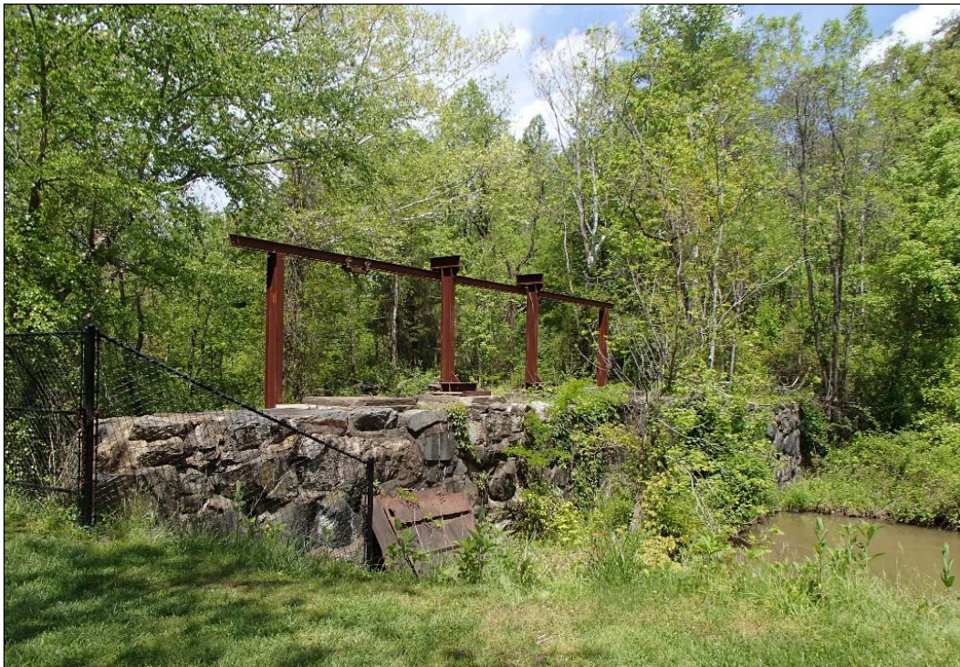
Figure 21: Altamahaw Cotton Mill, sluice gate, east elevation
