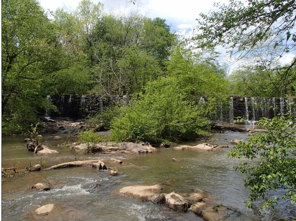
Figure 26: Altamahaw Cotton Mill, Haw River dam, east elevation
