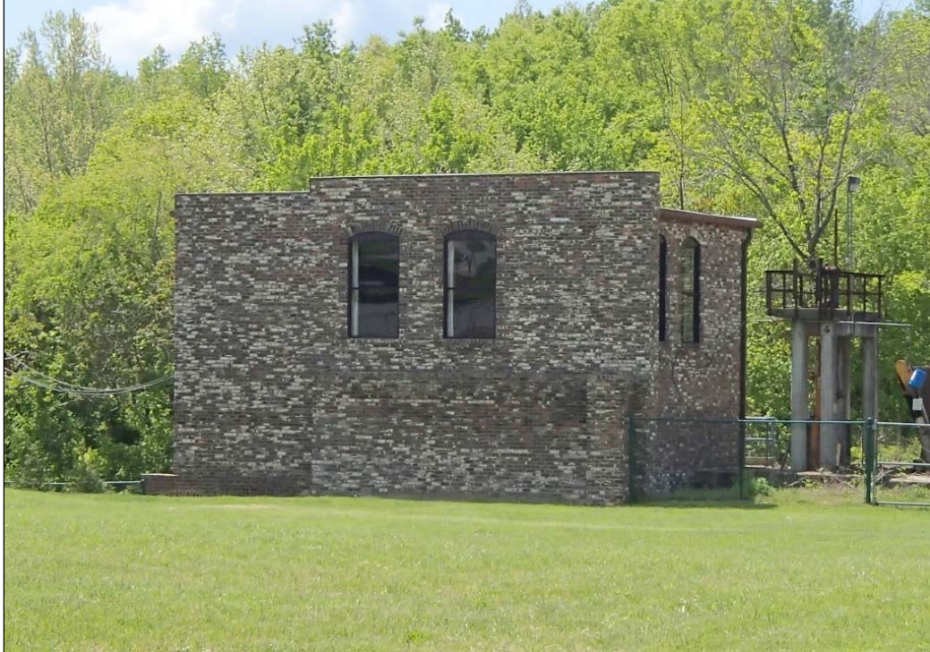
Figure 10: Altamahaw Cotton Mill, powerhouse, north elevation
