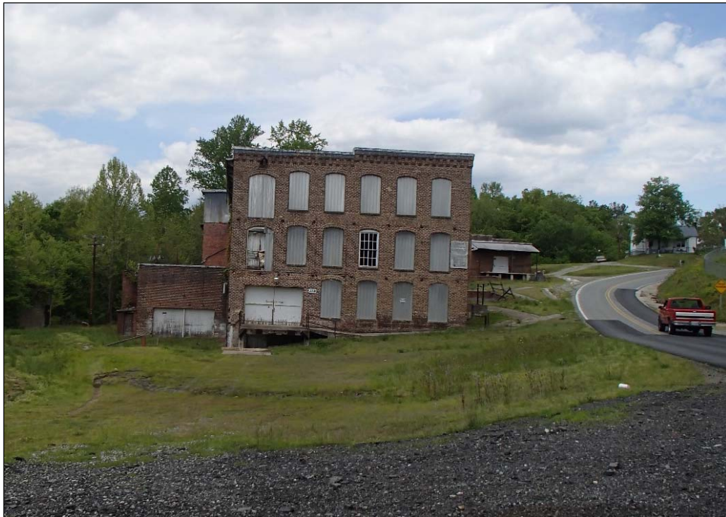
Figure 29: Carolina Mill, southeast elevation
