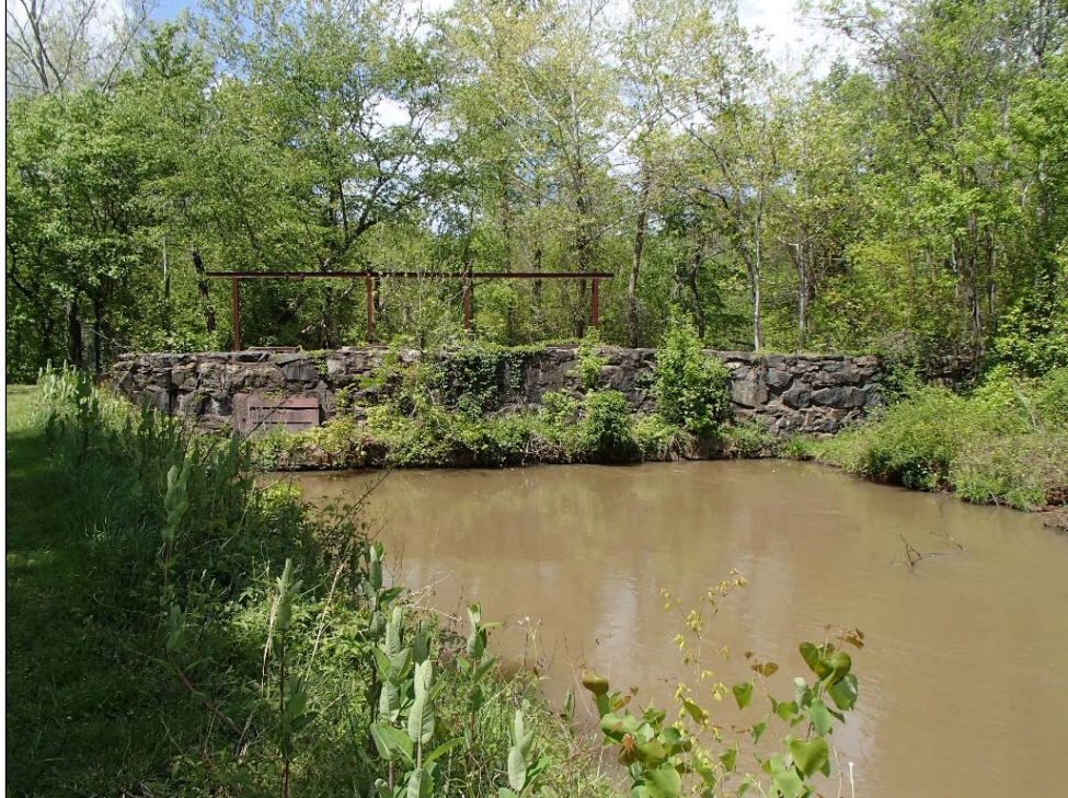
Figure 20: Altamahaw Cotton Mill, sluice gate, east elevation
