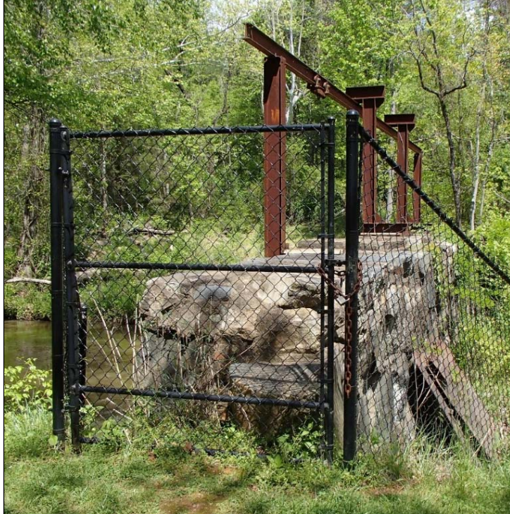
Figure 22: Altamahaw Cotton Mill, sluice gate, facing north
