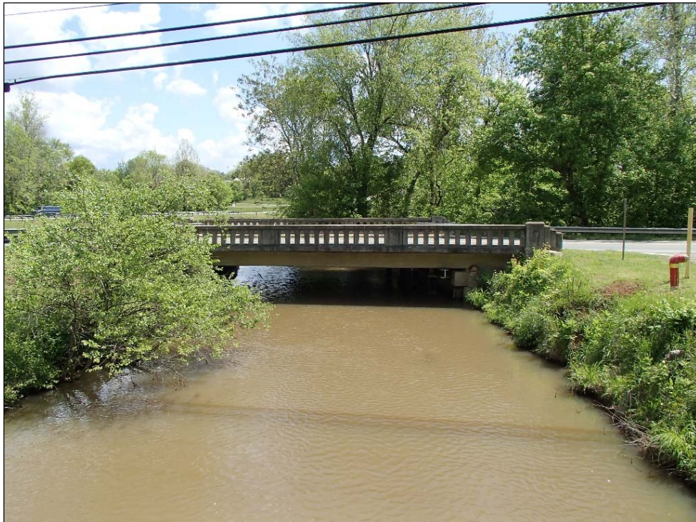
Figure 17: Altamahaw Cotton Mill, mill race and west side of Bridge No. 126
