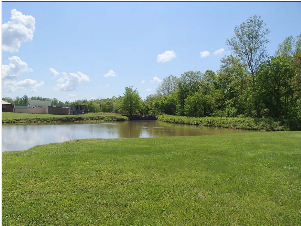
Figure 13: Altamahaw Cotton Mill, facing east toward 2nd sluice gate and power house
