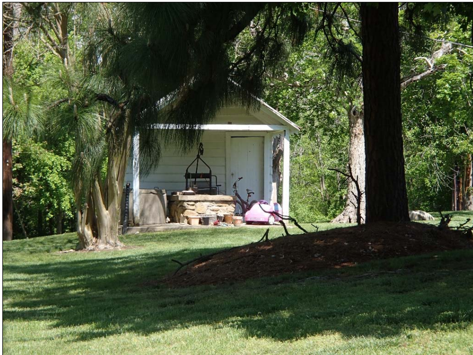
Figure 43: Simpson House, well house, south elevation
