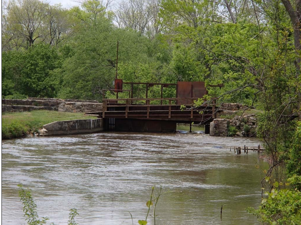
Figure 32: Glencoe Mill, sluice gate, southeast elevation
