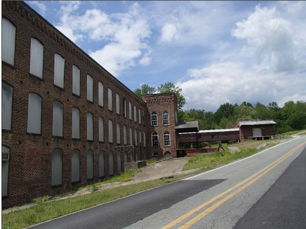
Figure 30: Carolina Mill, facing northwest
