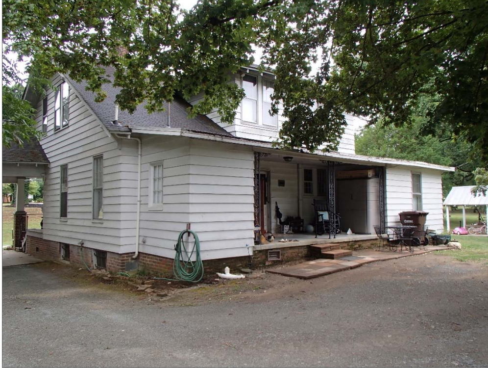
Figure 38: Simpson House, northeast corner
